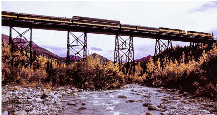
Riley Creek Railroad Bridge
