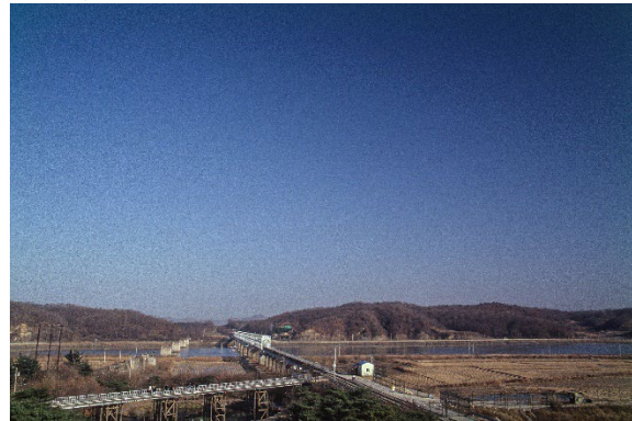
New Railroad Bridge to North Korea
